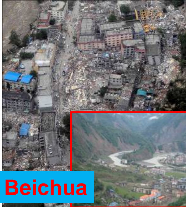
Collapsed houses after the earthquake
