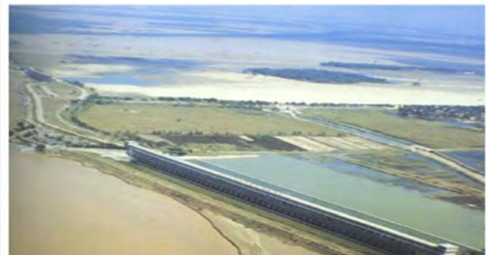
Flood intake gate in the Dongping Lake flood retention area of the Yellow River
