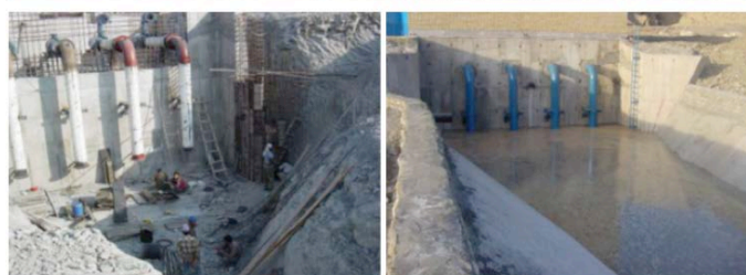
Emergency pumping station (bottom) to exploit dead storage of the Minab Dam (Top) located in Hormozgan Province (Southern Iran)
