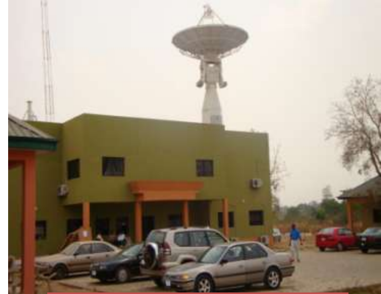
Ground Receiving Station
