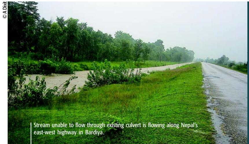
Stream unable to flow through existing culvert is flowing along Nepal's east-west highway in Bardiya.
