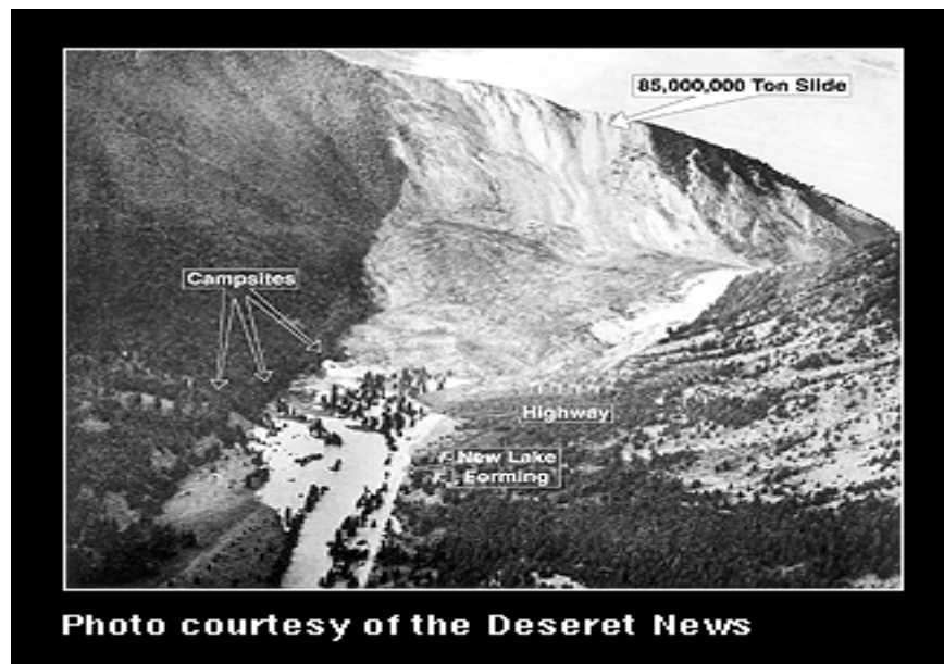
Figure 5.2 Landslide caused by Hebgen Lake Earthquake in 1959.
